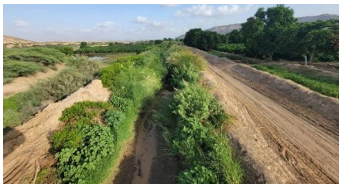
Before implementation | Photo Credit: UNDP Cleaning channels of trees and sediments, Imjila Al-Rahwi Batis
