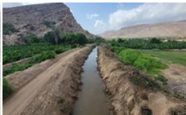
After Implementation | Photo Credit: UNDP Cleaning channels of trees and sediments, Imjila Al-Rahwi
